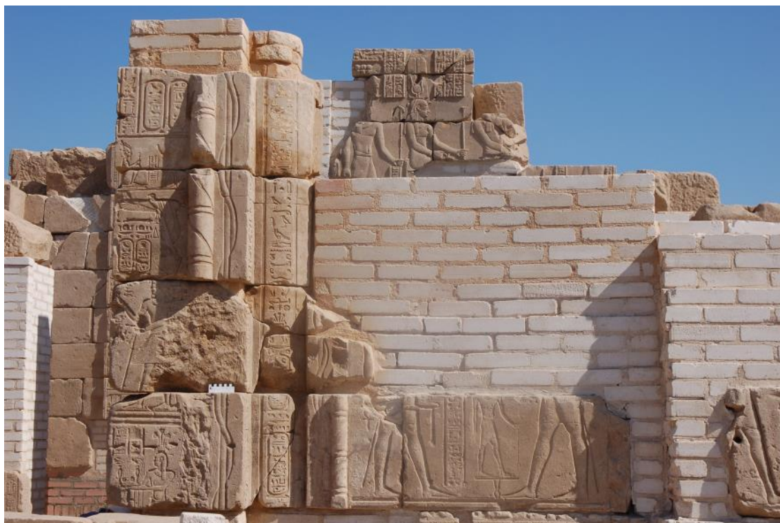
Fig. 35: Masonry completion of row next to the eastern column (photo: M. Fielauf © SIK).
