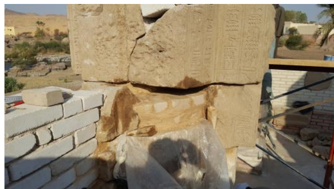
Fig. 34: Masonry completion of row 3 of the eastern column (photo: M. Fielauf © SIK).
