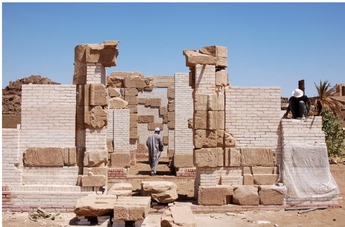
Fig. 31: Façade of Nesmeti temple after final positioning of blocks (photo: C. von Pilgrim © SIK).
