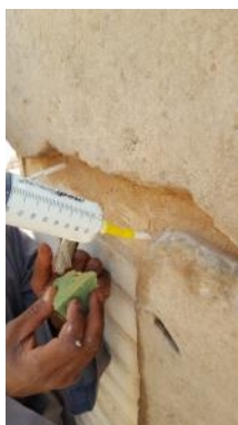
Fig. 33: Filling smaller cracks and joints with Ledan TA1 (photo: M. Fielauf © SIK).
